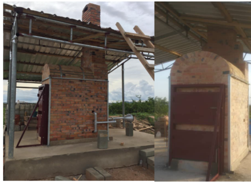
Figure 5. The modified De-Montfort type incinerator [50].
