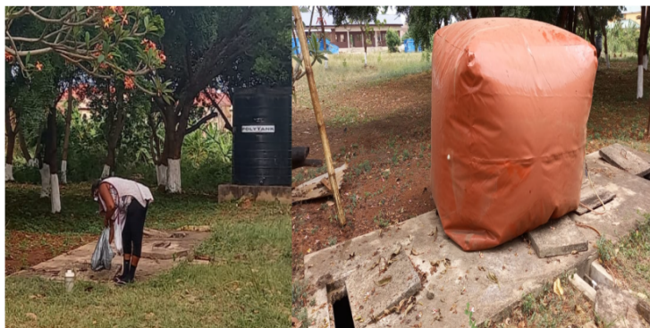
Figure 3. Manual feeding of the biodigester with food waste and gas collected in a balloon.
